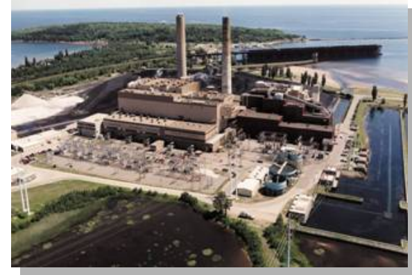
Combustion Power Plant
