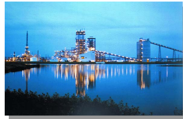
IGCC Power Plant
